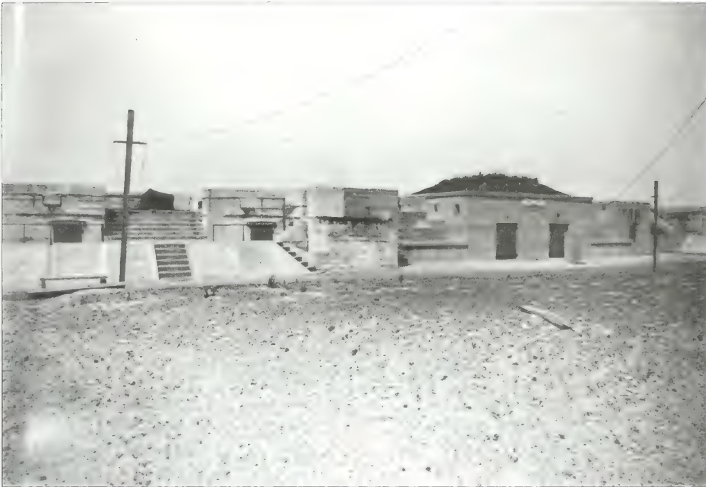
Figure 5.21. View looking northeast at Battery Urmston, circa 1900. In contrast to its appearance today, the south side of Battery Urmston contained no woody vegetation (GATE 7882).
